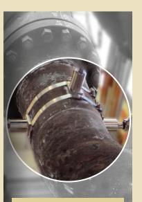
INSTALLATION Unit sensors are mounted on the prepared surface.
