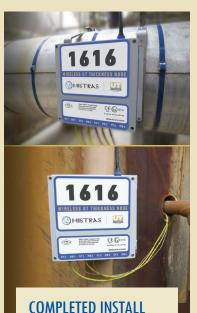
System mounted and installed on horizontal (top) and vertical (bottom) piping.
