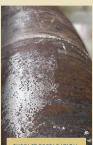
SURFACE PREPARATION Ground clean to prepare the surface where the 1616 node will be installed for use.
